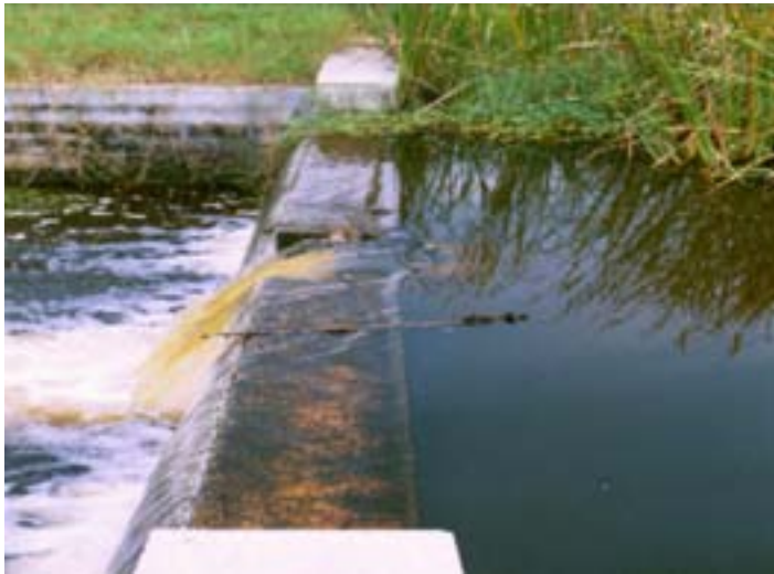
Figure 14. Weir structure used as outfall from water detention area.
