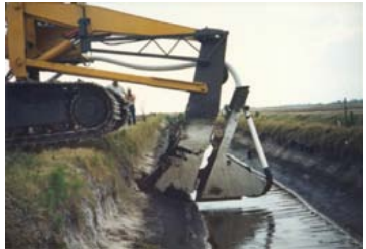
Figure 19. Installing 4-inch corrugated drain tubing with PVC pipe discharge.
