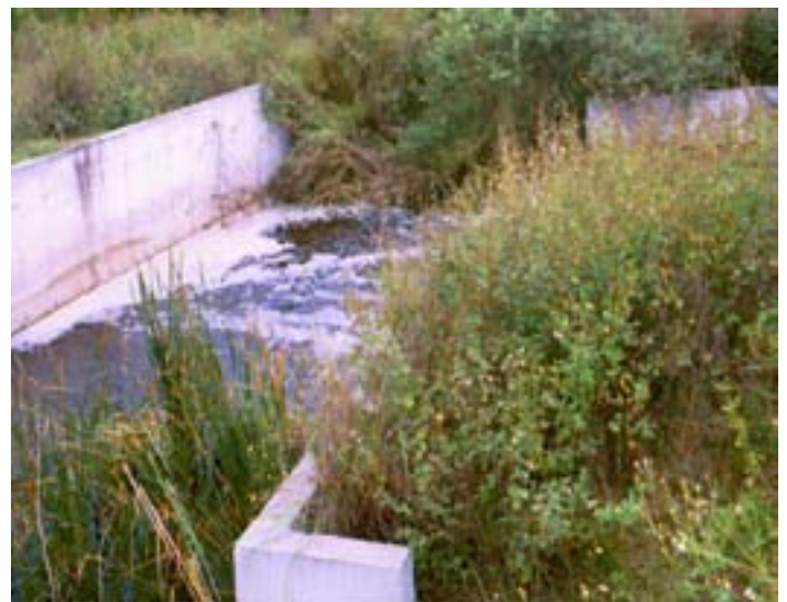
Figure 16. Erosion control structure on grove discharge canal.
