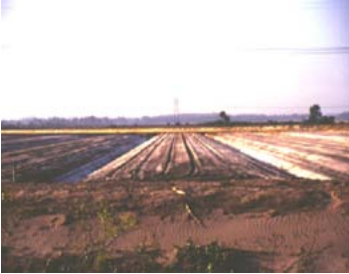
Figure 9. Double-row bed under construction.
