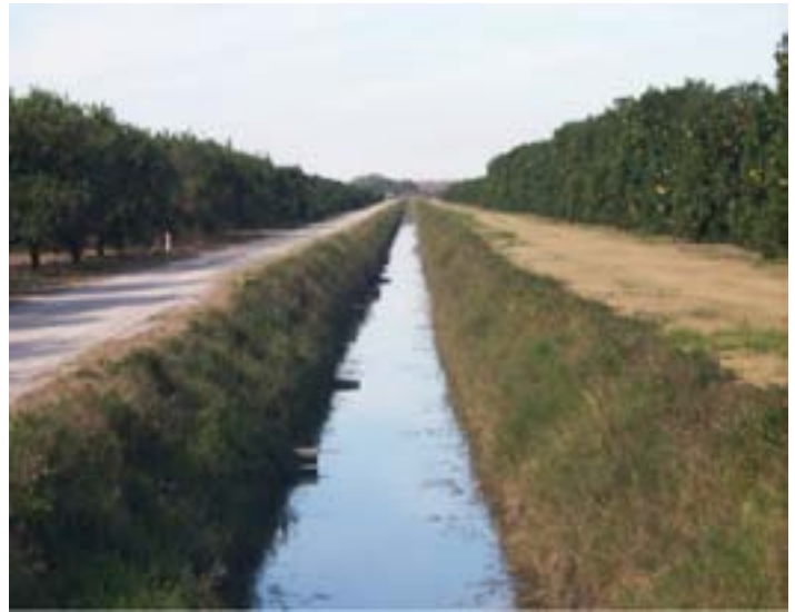
Figure 11. Lateral drainage ditch with water furrow outlet pipes discharging into ditch.
