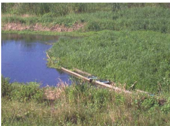
Figure 5. Hyacinth barrier installation. Credits: P. Whalen
