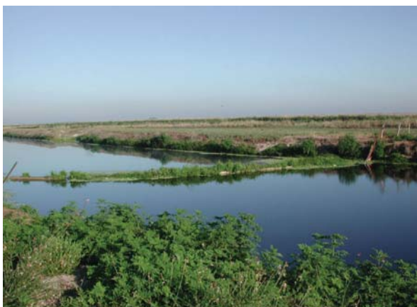
Figure 4. Ribbon barrier installed on canal. Credits: P. Whalen
