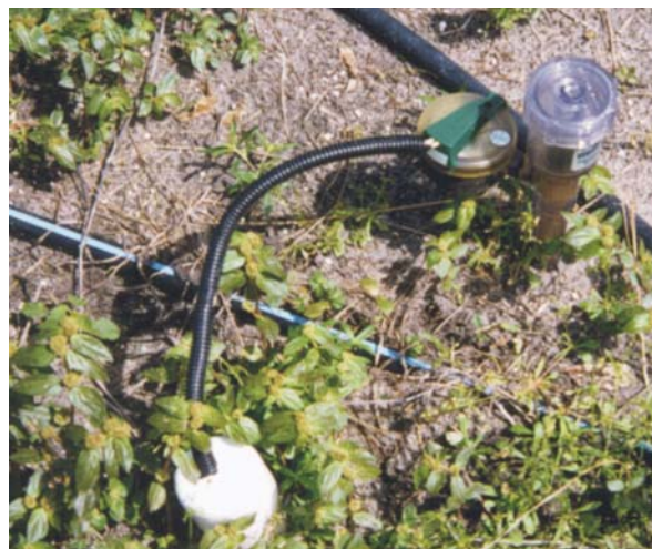
Figure 1. Switching tensiometer used to control irrigation system in microirrigated citrus grove.
