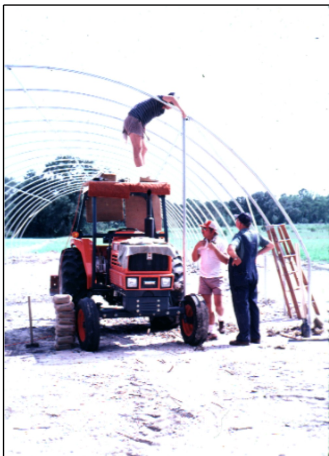
Figure 1. Greenhouse under construction.
