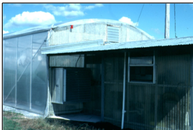
Figure 3. "Airlock" entrance porch to minimize entry of pests into greenhouse.
