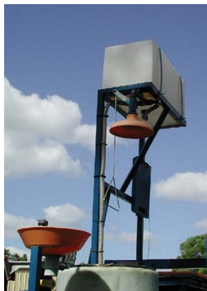
Figure 3. Portable mix-load stations: closeup of eyewash and shower.
