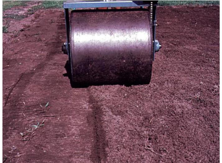
Figure 2. Final Grading
