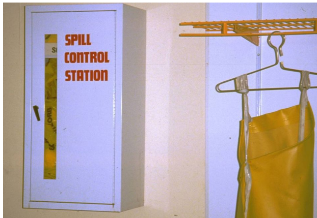
Figure 1. Permanent-sited spill kit cabinet.
