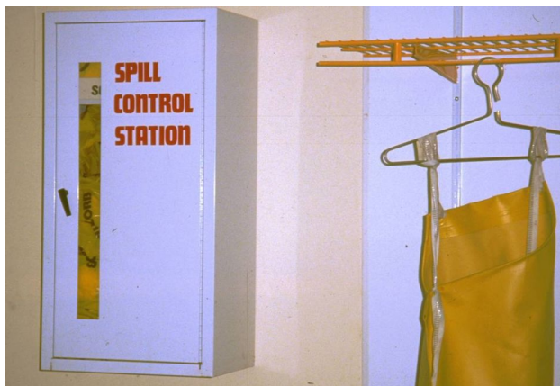
Figure 1. Permanent-sited spill kit cabinet.
