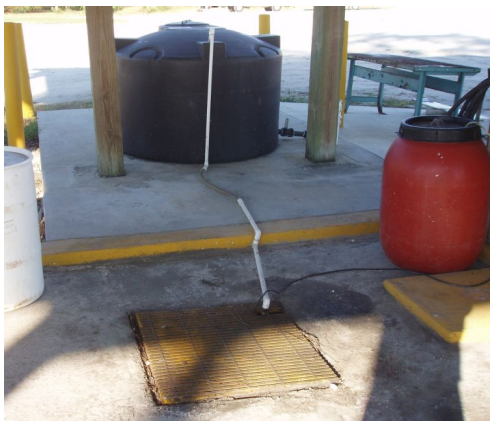
Figure 5. Containment Pad and Tank for Holding Wastewater Credits: UF/IFAS Pesticide Information Office
