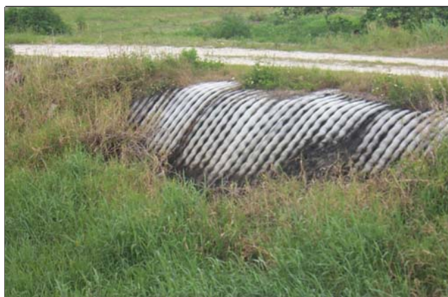
Figure 5. Canal bank stabilization in a high velocity area using a hardened synthetic ground covering. Credits: PCW
