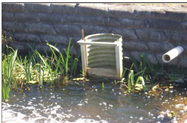
Figure 4. Stabilization of a grove crossing with concrete wall structures. Credits: PCW
