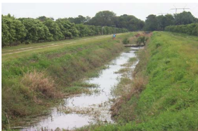
Figure 2. Well maintained vegetation on ditch side-banks. Credits: PCW
