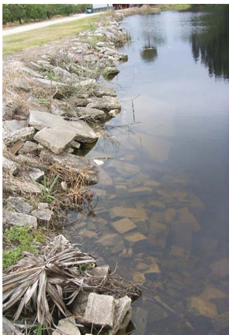
Figure 3. Ditch side-bank stabilization using broken concrete refuse. Credits: PCW
