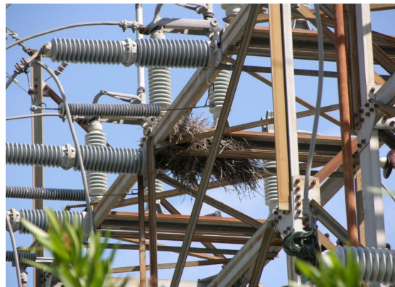
Figure 1. Monk Parakeets build huge, communal nests on power distribution stations. When wet, these nests can disrupt power, and they are costly (and dangerous) to remove. Credits: Steve A. Johnson
