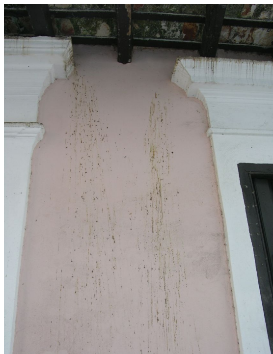
Figure 2. European Starlings, Eurasian Collared-doves, Rock Doves, and other introduced birds nest and roost on buildings. They produce large amounts of feces that can corrode or stain walls and is difficult to remove. Credits: Steve A. Johnson
