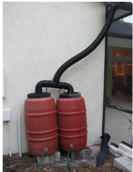
Figure 2. Good linked barrel design, but not level. Credits: Lynn Barber, UF/IFAS
