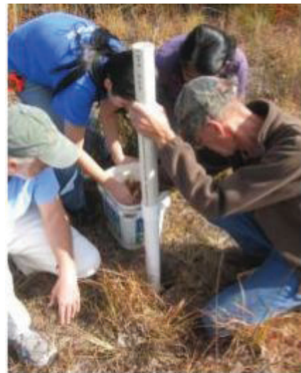
Figure 1. Citizen scientist volunteers assist in the installation of groundwater monitoring wells. Credits: L. Gommerman.
