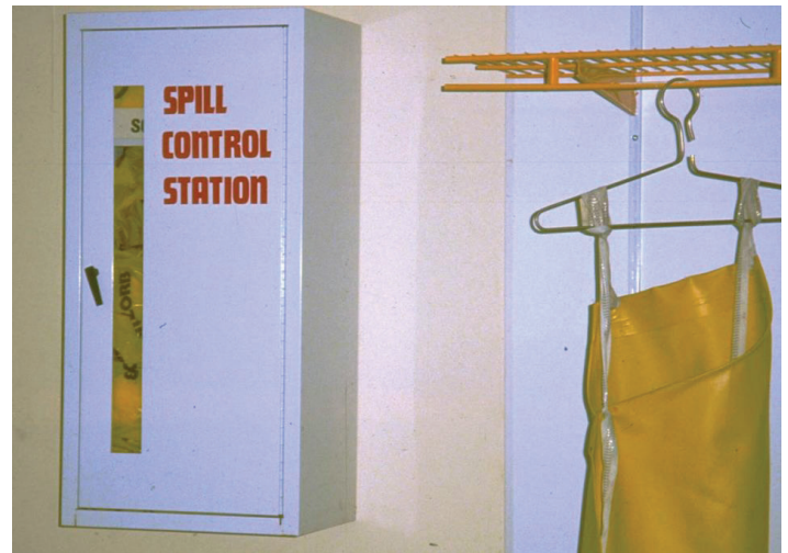
Figure 1. Permanent-sited spill kit cabinet. Credits: UF/IFAS
