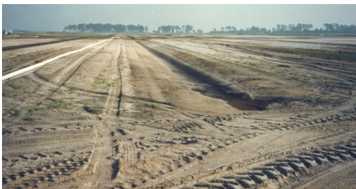
Figure 2. Typical construction of 2-row beds in flatwoods citrus groves.
