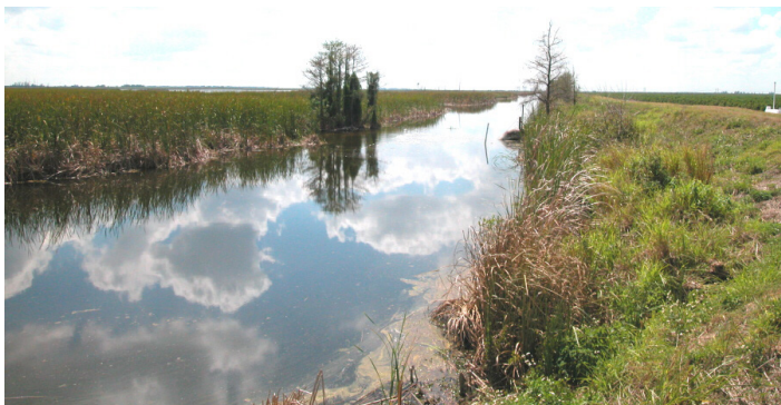
Figure 1. Berm and interior of typical retention/detention area within citrus grove.
