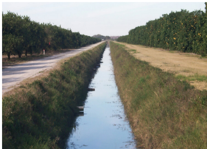
Figure 3. Typical lateral ditch and water furrow pipe configuration in flatwoods citrus groves.
