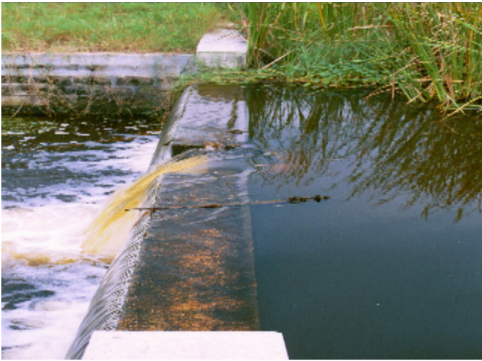
Figure 7. V-notch weir outfall on citrus wet detention area.
