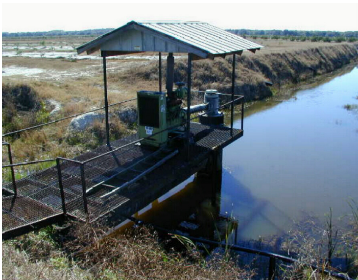
Figure 4. Drainage pump on flatwoods citrus grove collector ditch.
