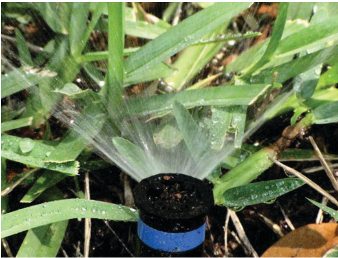
Figure 3. Standard head with a fixed spray nozzle. Credits: Bernard Cardenas, UF/IFAS
