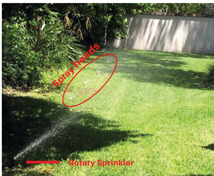
Figure 2. Mixed sprinkler types. Note: Rotary sprinkler in foreground and spray heads in background. Credits: Bernard Cardenas, UF/IFAS
