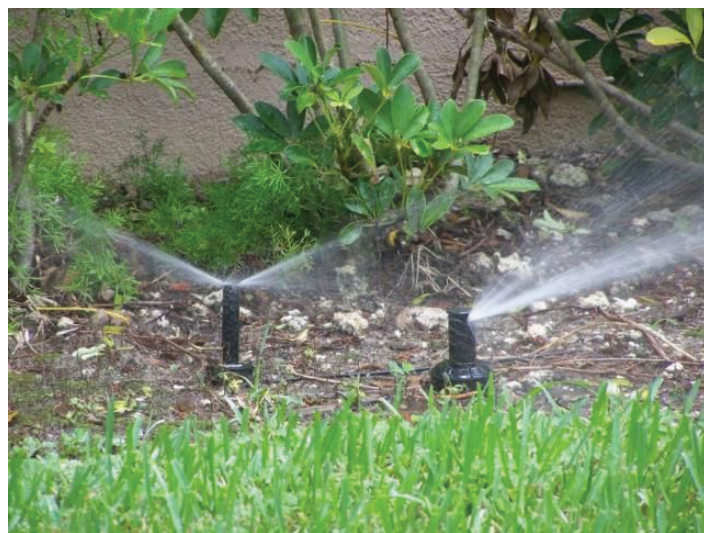
Figure 1. Ornamentals and turfgrass being irrigated from the same irrigation zone. Note: The spray head in the background is irrigating the ornamentals and the rotary sprinkler is irrigating the turfgrass in the foreground.
