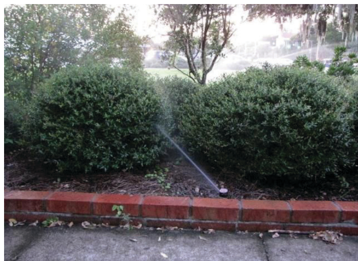
Figure 3. Blocked water spray. Credits: Bernard Cardenas, UF/IFAS
