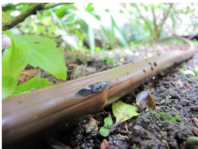
Figure 4. Drip tubing in-line emitter. Credit: Michael Gutierrez, UF/IFAS
