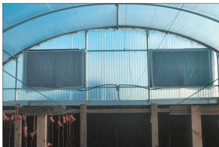
Figure 9. Inside photo of motorized shutters covered with insect exclusion fabric.
