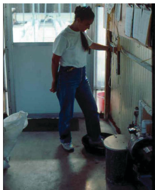
Figure 13. Entrance air-lock porch provides space for foot bath for sanitation purposes.
