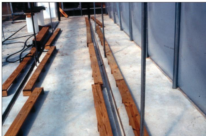
Figure 20. Drainage troughs created by pouring concrete floor around wooden forms and then removing forms, leaving behind troughs. Wooden benches also shown in photo.
