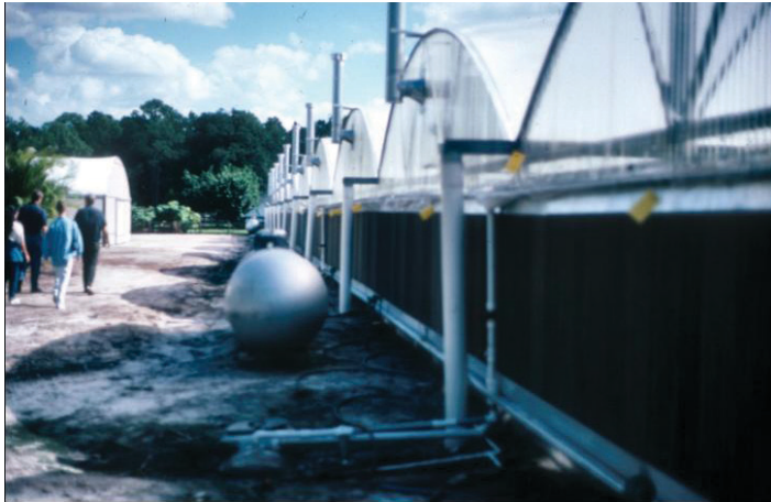
Figure 10. Evaporative cooling pad with underground water return system.
