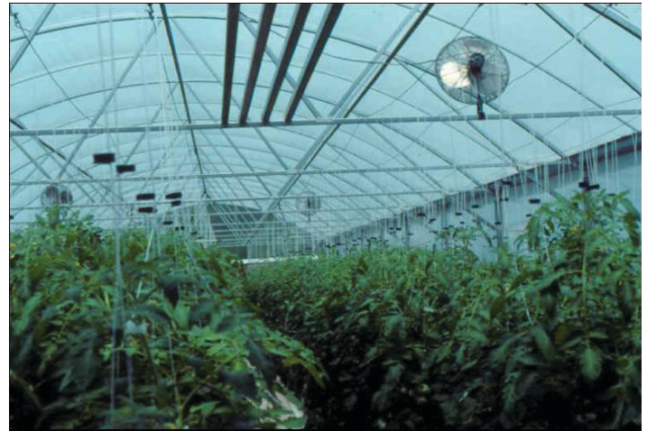
Figure 22. Horizontal air-flow fans. Credits: UF/IFAS
