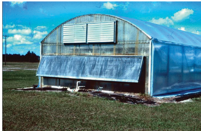
Figure 8. Cooling-pad endwall with open area for evaporative pad (in this photo, covered with motorized shutter) and 2 openings for motorized shutters, above cooling pad.
