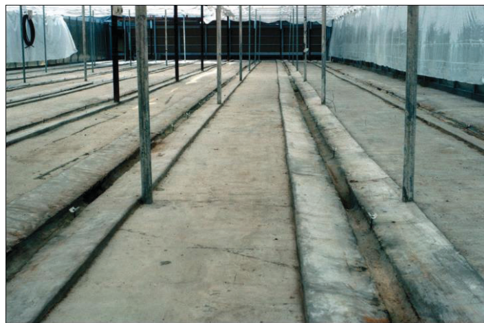
Figure 18. Concrete slanted pads for drainage leachate.
