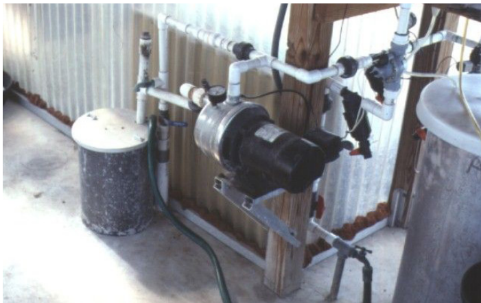
Figure 6. NFT recirculation pump and sump tank (note raised-neck opening to sump tank) Credits: UF/IFAS
