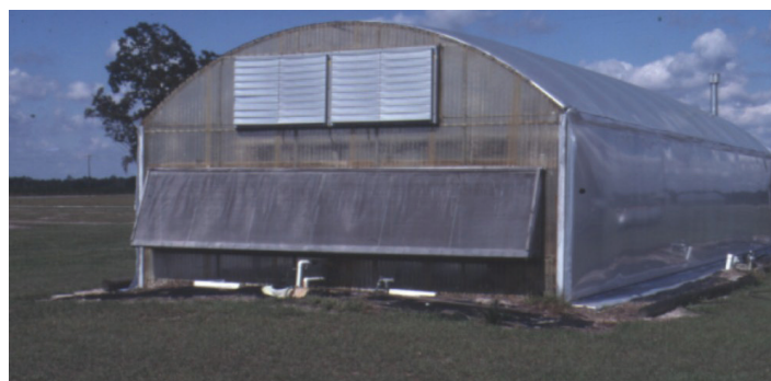
Figure 30. Motorized inlet shutters for winter ventilation.
