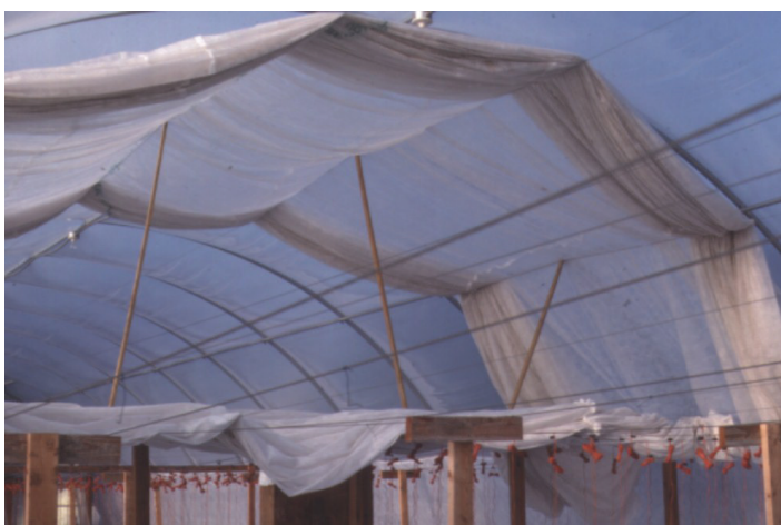
Figure 31. Greenhouse ceiling contour shade cloth system.
