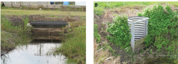
Figure 6. An example of two types of riser-board control structures present on aquaculture facilities in Florida. The image on the left (A) shows a concrete structure with visible riser boards while the image on the right (B) shows a less expensive alternative using galvanized steel pipe.
