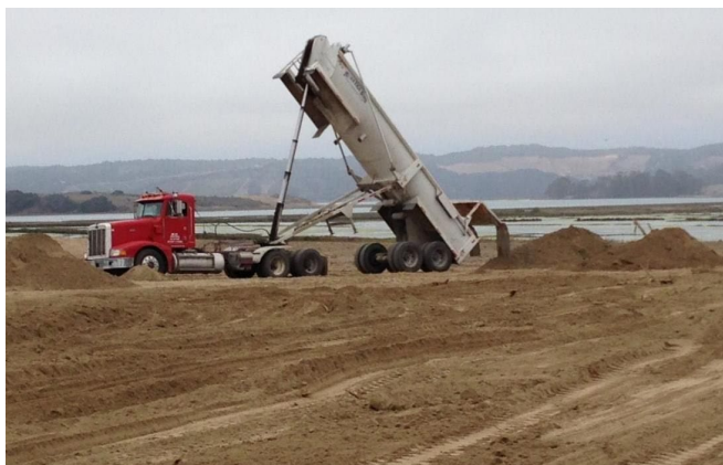
Figure 6. Construction equipment placing and spreading sediment for thin layer placement at a salt marsh restoration site in Elkhorn Slough, California.
