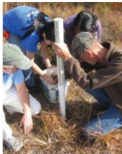
Figure 1. Citizen scientist volunteers assist in the installation of groundwater monitoring wells. Credits: L. Gommerman.
