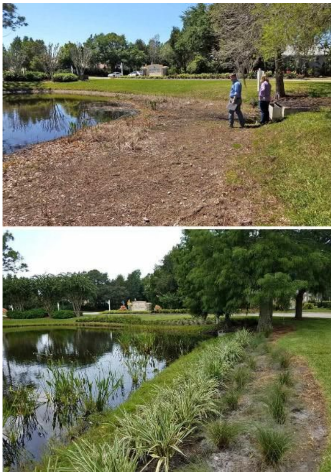
Figure 2. Before (top) and after (bottom) stormwater pond plantings. The pond on the left is more likely to experience soil erosion and nutrient-rich grass clippings entering the water, both of which can degrade water quality via increasing nutrient levels.
