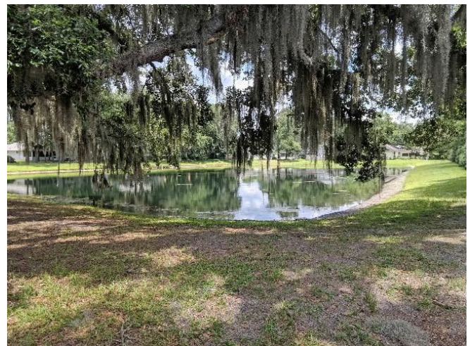
Figure 1. A typical stormwater pond in a Florida community. Note the bank erosion and lack of plantings along its perimeter.
