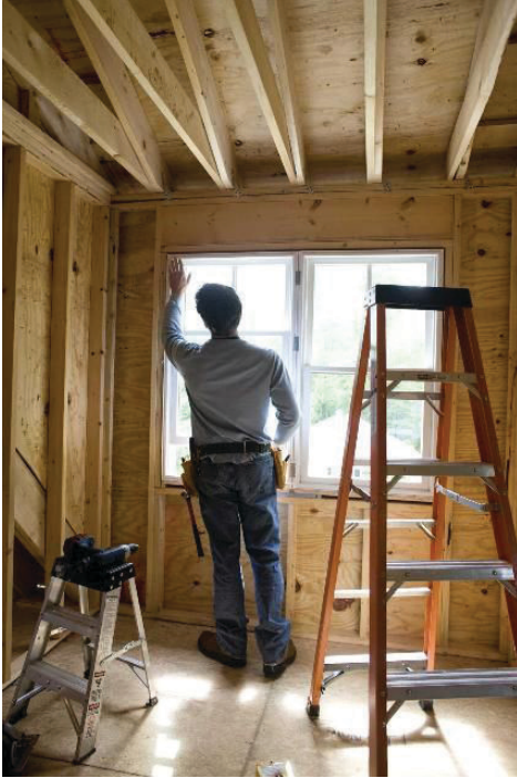
Figure 1. You should carefully consider the selection of contractors prior to allowing them to work on your home, to ensure you understand the hiring process and agree on specific details before signing a contract.
