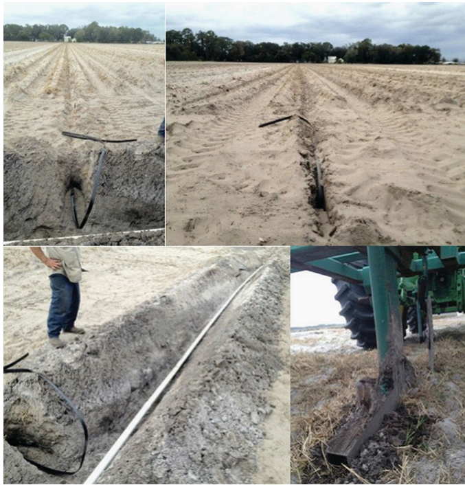
Figure 7. Installation of subsurface drip tape at a depth of 24 in. below the soil surface in a potato field, Hastings, Florida. Upper figures: subsurface drip tape positioning after the installation. Lower left: detail of the manifold (PVC). Lower right: chisel plow adapted for subsurface drip installation.
