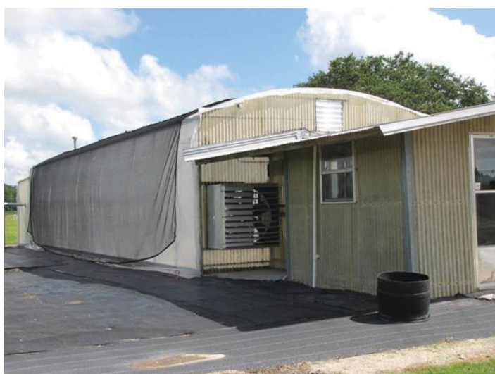
Figure 3. Fan and pad type ventilated greenhouse. Credits: UF/IFAS
