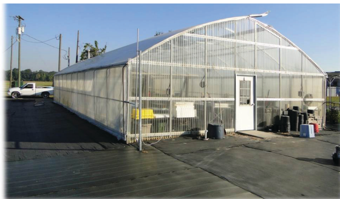
Figure 4. Passively ventilated greenhouse structure. Credits: UF/IFAS
