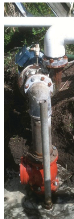
Figure 1. The 2" drop pipe (galvanized) installed below red check valve of original 6" well.
