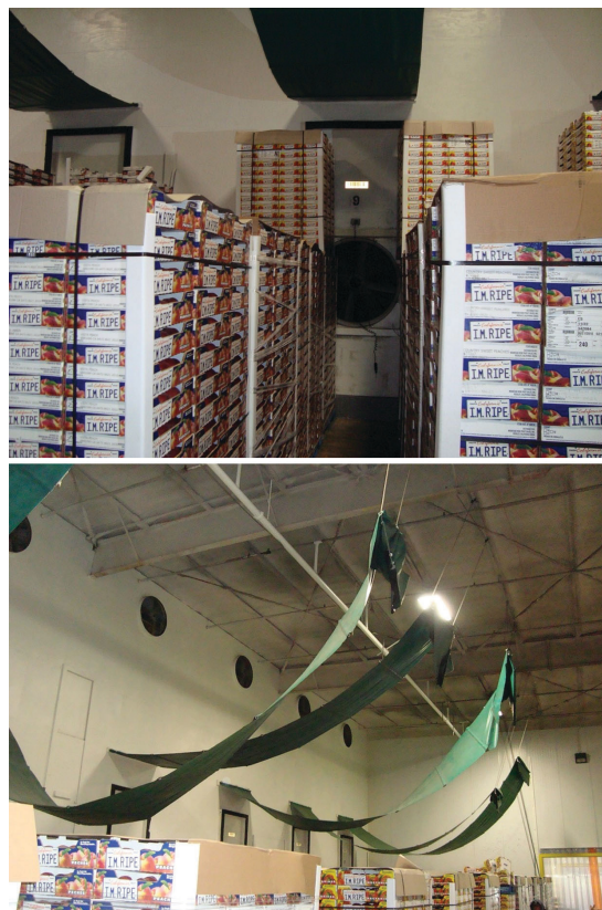
Figure 8-5. Forced-air cooling of peaches in palletized shipping cartons. The pallets have been aligned in rows on either side of fans set into the cold room wall to form the cooling tunnels, prior to lowering the tarps and turning on the fans to begin forced-air cooling. Credits: Jeffrey K. Brecht, UF/IFAS
