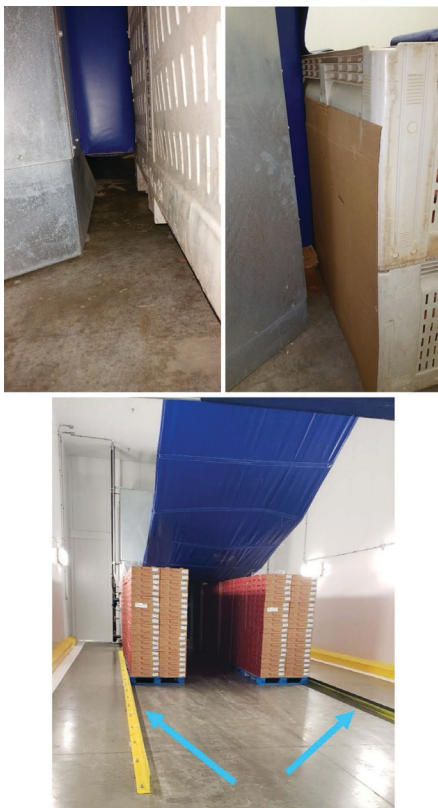
Figure 8-6. Side view at the front of a forced-air cooling tunnel showing: (top left) openings under blue foam pad and at the base of the white adjoining bin; and (top right) these openings blocked with corrugated sheets to improve cooling efficiency. In the bottom image, the fixed angle irons serve to align the pallets as well as block airflow underneath the pallets.
