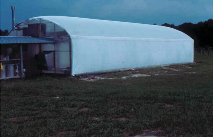
Figure 26. Greenhouse with woven shade cover.
