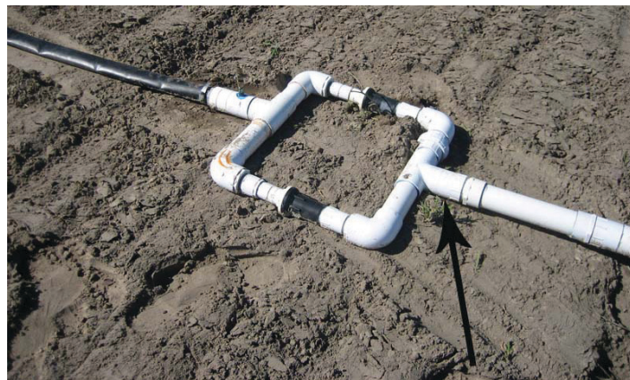
Figure 7. Pressure regulators are installed side-by-side in this system to allow a greater flow rate. Note the small injection port for chemical injection. Credits: Eric Simonne.
