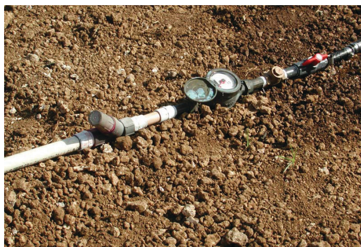
Figure 8. Water meters installed near the field. Credits: Eric Simonne.
