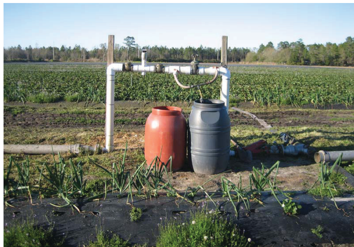
Figure 4. Back-flow prevention made of two ball valves and a vacuum breaker are placed upstream of the Venturi injector. Credits: Eric Simonne.
