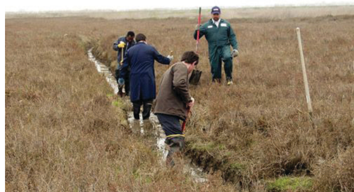
Figure 15. Mosquito control professionals digging a drainage ditch for mosquito source reduction.
