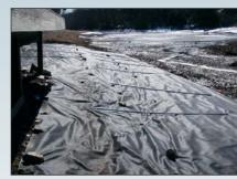
Figure 21. Benthic barrier (Aquascreen®) installed after a drawdown. Photograph by Matthew Vogt, New England Aquatic Services LLC.
