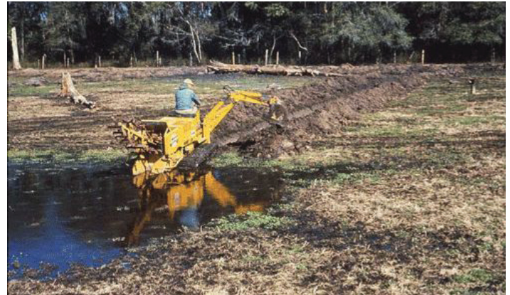
Figure 11. Digging drainage canals to remove standing water is one method to reduce mosquito larval developmental opportunities.
