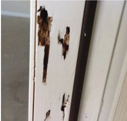
Figure 2. Termite damage on a door frame. Door frames are common access points. Doors often sit on expansion joints that allow subterranean termites to find their way in. Credits: Faith Oi, UF/IFAS
