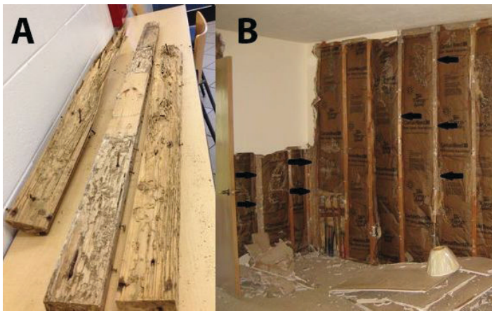
Figure 31. A) Subterranean termite damage in a room; B) Termites are blind, soft-bodied insects, so they follow guidelines, including wall studs. Arrows denote areas of prominent mud tubes. Credits: Faith Oi, UF/IFAS
