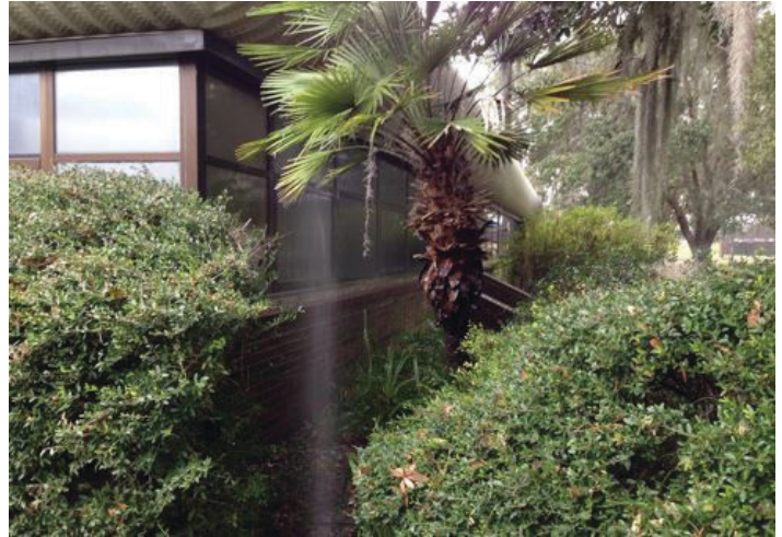
Figure 12. Irrigation head improperly directed, resulting in walls being watered. Wet walls create a conducive condition that will allow termites to thrive. Credits: Faith Oi, UF/IFAS
