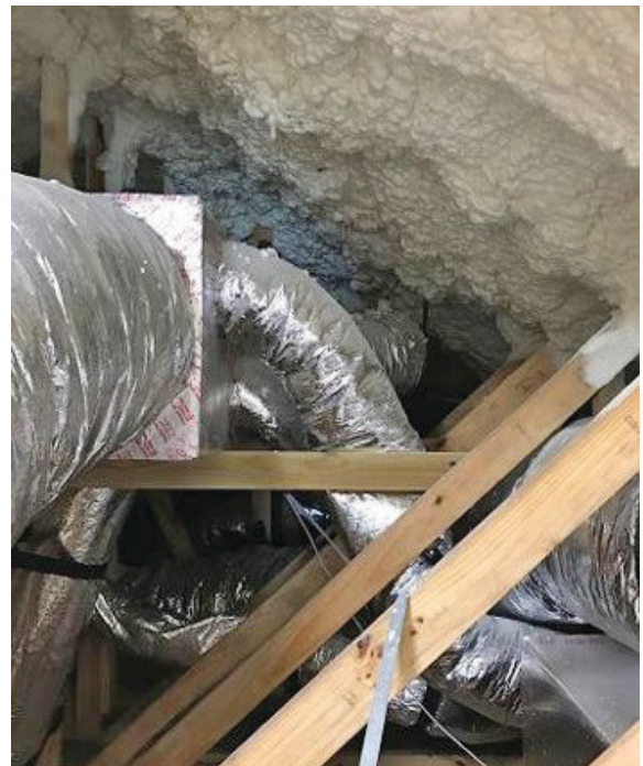
Figure 5. Spray foam insulation that obscures inspections and duct work that makes this space inaccessible for inspections. Credits: Faith Oi, UF/IFAS
