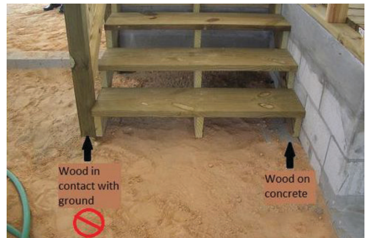
Figure 9. Example of wood-to-ground contact. Other examples in homes that may have wood-to-ground contact include piers, posts, attached fences, and decks. In this picture, the part of the wooden stair that is on the concrete pad may gain slightly more protection, but termites can still find the stairs via the gap against the wall. Credits: Faith Oi, UF/IFAS
