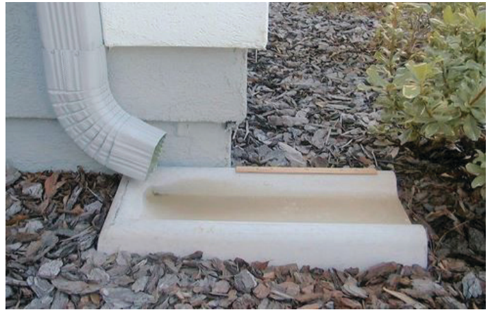
Figure 13. Splash block to divert water from gutter away from home. Credits: Faith Oi, UF/IFAS
