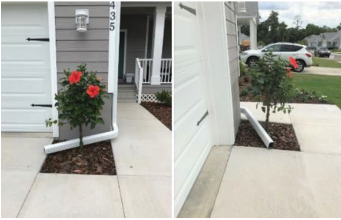
Figure 15. Improper plant placement and poor gutter placement. This newly planted hibiscus is one foot away from the home, but the branches are already almost touching the wall.
