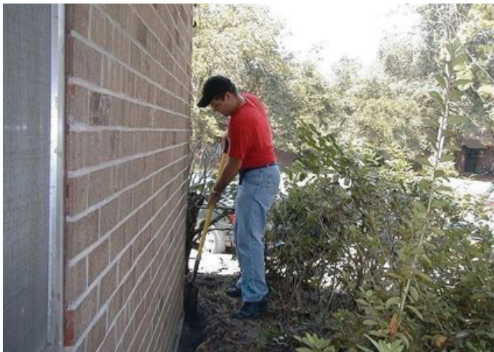
Figure 34. Trenching so that the termiticide can be applied into the trench according to the product label rate to cut off subterranean termite access from the outside.
