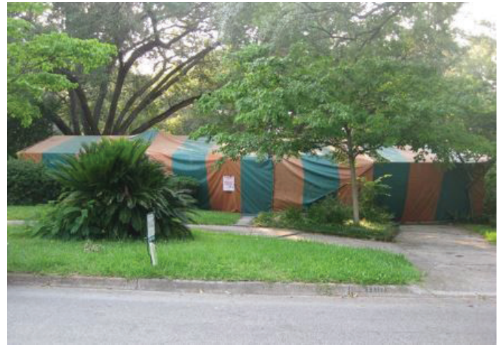
Figure 25. Fumigation is highly effective against drywood termites. Structures are tented and tightly sealed to hold the fumigant (active ingredient: sulfuryl fluoride). It is critical that no one enter the structure because the gas is highly toxic. Once properly aerated and cleared using sensitive instrumentation, the home can be entered again.
