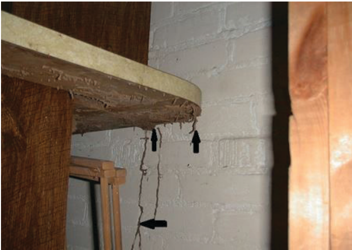
Figure 27. Subterranean termite mud tubes on wall and under countertop. Credits: Faith Oi, UF/IFAS
