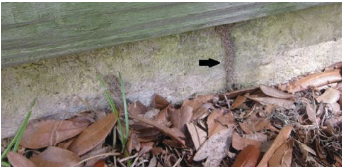
Figure 11. Termite tube that was detected on outside foundation wall that had an inspection space. Credits: Faith Oi, UF/IFAS
