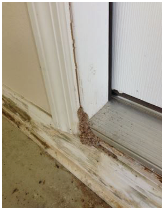
Figure 30. Subterranean termite mud tube at garage door baseboard and door frame, a common entry point. Credits: Faith Oi, UF/IFAS
