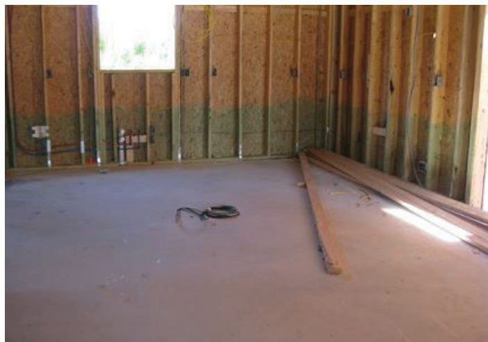
Figure 39. Borate-treated wall with a dye marker that shows where the treatment was applied.
