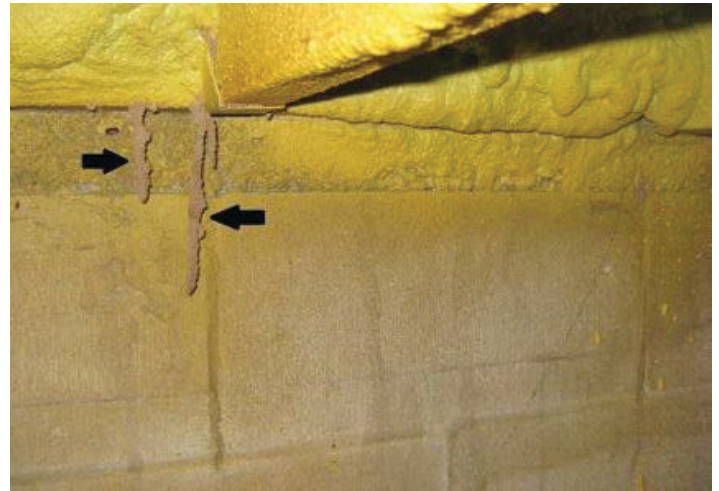
Figure 4. Arrows denote subterranean termite mud tubes emerging from behind spray foam insulation installed over floor joists in crawlspace. Credits: Faith Oi, UF/IFAS
