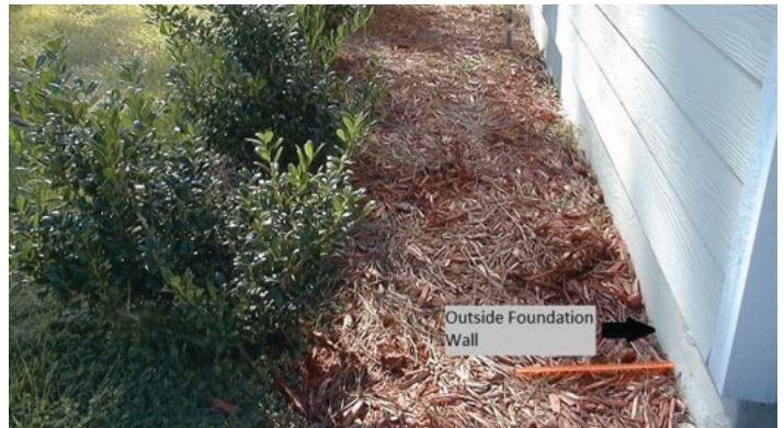
Figure 14. This home has maintained an excellent inspection space between the siding and mulch. Landscape plants are also positioned far enough away from the outside foundation wall to decrease moisture close to the home, and the placement accounts for future growth. Moisture is a conducive condition that can void some termite warranties. Credits: Faith Oi, UF/IFAS
