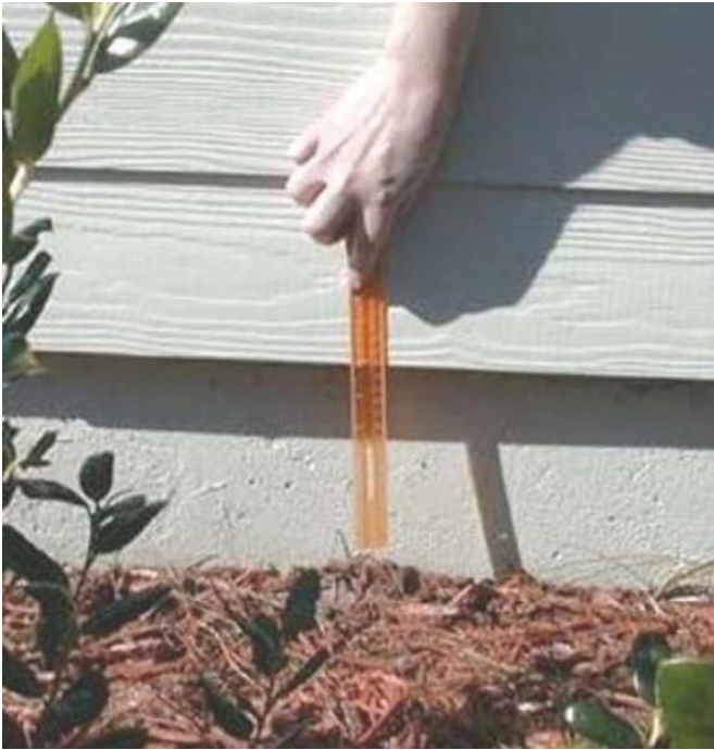
Figure 10. Building codes in many states require at least a 6-inch inspection space at the time of construction. It is important to maintain this inspection space and not hide it with mulch. When inspection spaces are obscured by mulch or other landscape plants, subterranean termites can access structures. Credits: Faith Oi, UF/IFAS
