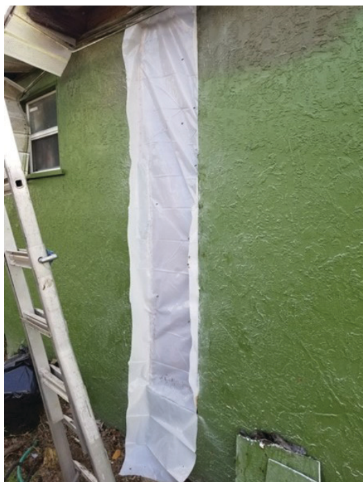
Figure 14. Unless you are a licensed and insured contractor, you should not attempt to repair a structure yourself. Flexible plastic sheeting can be used to provide a temporary seal. Credits: Jason Deeringer, Bee Serious Bee Removal, LLC
