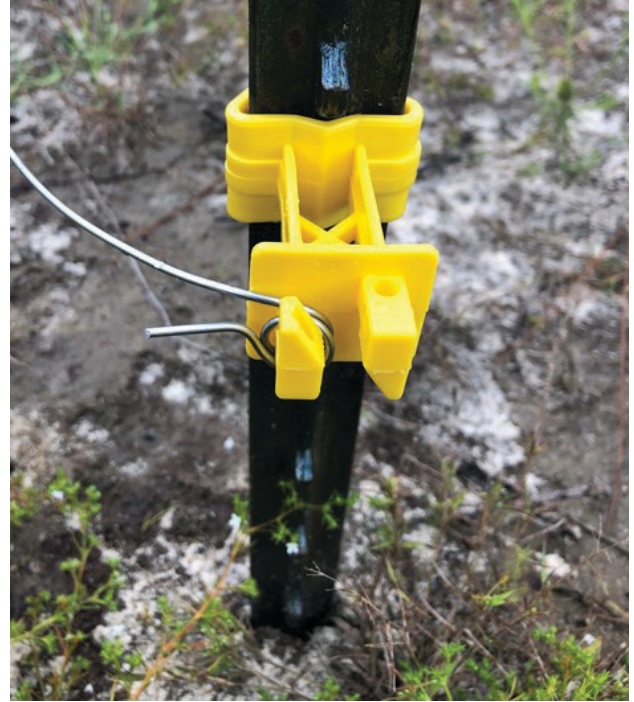
Figure 5. Wrap wire at first insulator. Credits: K. Post, UF/IFAS
