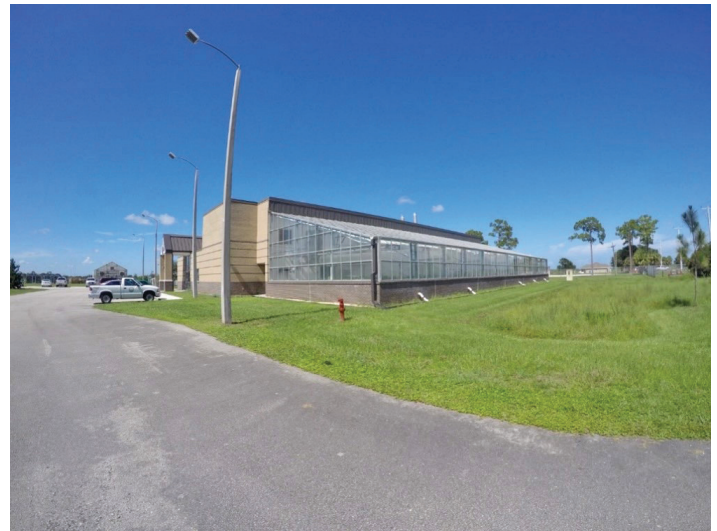
Figure 3. UF/IFAS Hayslip Biological Control Research and Containment Laboratory, a USDA-APHIS inspected containment facility in Fort Pierce, FL that allows for the safe testing of arthropod biological control agents for weeds or arthropods. Credits: Carey R. Minter, UF/IFAS
