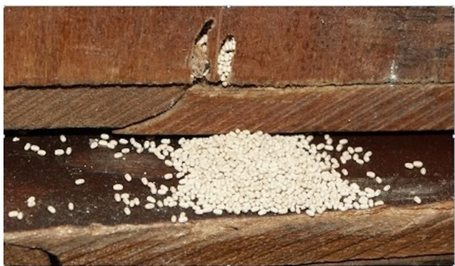
Figure 13. Pile of fecal pellets from Cryptotermes brevis (Walker).
