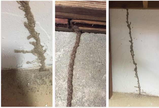
Figure 11. Foraging tubes (also called “mud tubes”) of the Formosan subterranean termite, Coptotermes formosanus . Credit: Aaron Mullins, UF/IFAS
