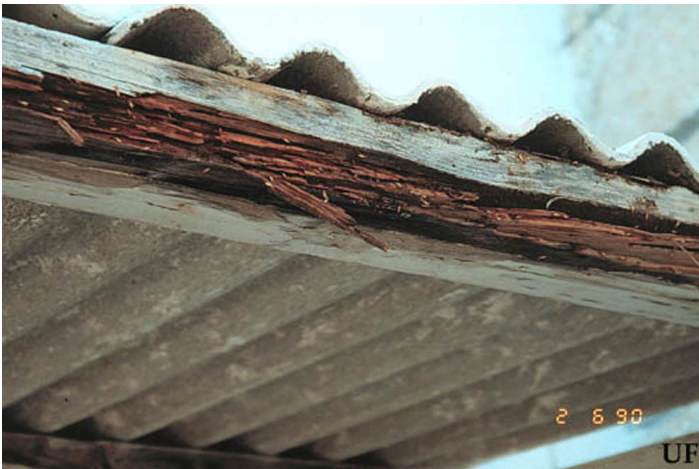
Figure 8. Damage by Coptotermes gestroi (Wasmann) to fascia, Grand Turk Island.
