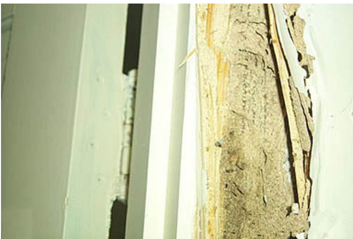
Figure 10. Carton material in door casing damaged by Coptotermes gestroi (Wasmann), Key West.
