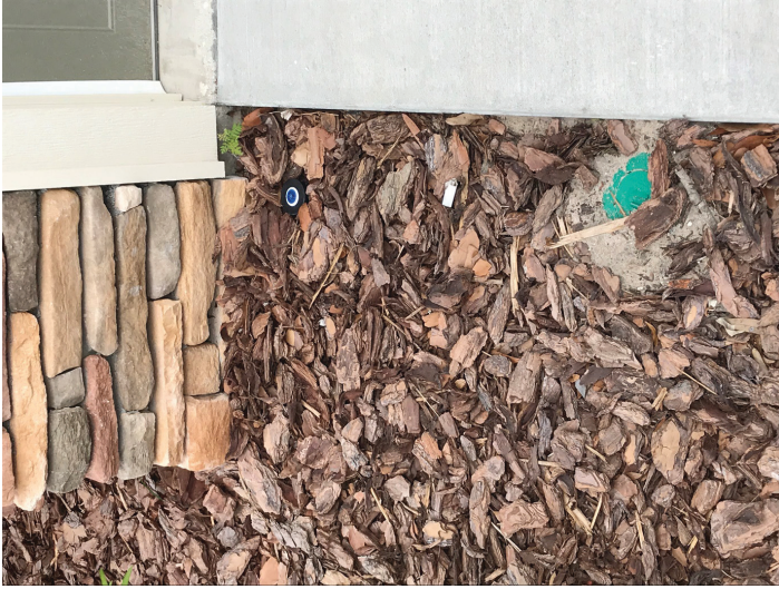
Figure 2. Faux rock is a popular wall covering. Pine bark mulch is covering the inspection space along the concrete slab combined and irrigation installed too close to the wall in violation of the current building code. The Florida building code requires that irrigation be installed 1 foot or more away from a building sidewall. Irrigation that “water walls” is considered a conducive condition that can void termite control warranties. There is enough moisture for weed growth. A termite bait was wisely installed in this area.
