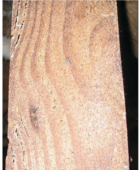
Figure 10. Damage on wooden pillar caused by larvae of the lesser mealworm, Alphitobius diaperinus (Panzer).
