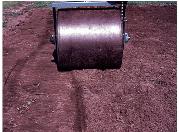
Figure 2. Final Grading
