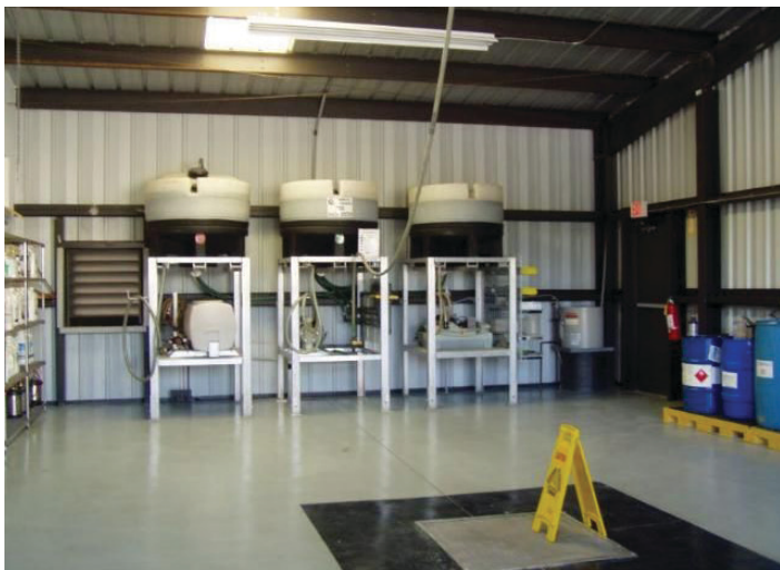
Figure 14. Rinse water can be re-used as make-up water in some cases. Credits: UF/IFAS Pesticide Information Office
