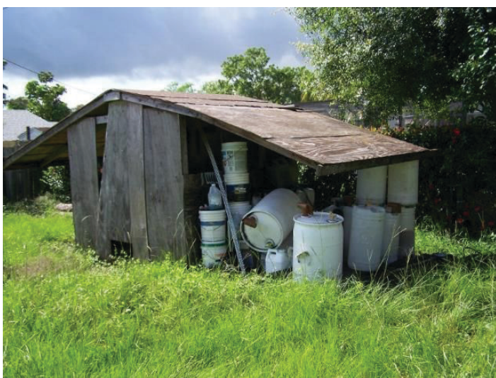
Figure 17. Excess drums pose a special disposal concern. Credits: courtesy of Florida Department of Environmental Protection
