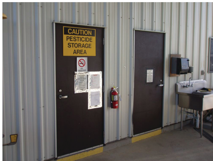
Figure 2. Example of a secure, well-marked storage facility. Credits: UF/IFAS
