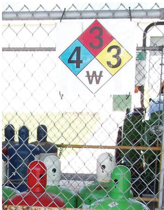
Figure 3. National Fire Protection Association warning at a fumigant storage site. The strikeover on the letter "W" in the white diamond alerts firefighters not to use water to put out a fire. Credits: F. M. Fishel, UF/IFAS
