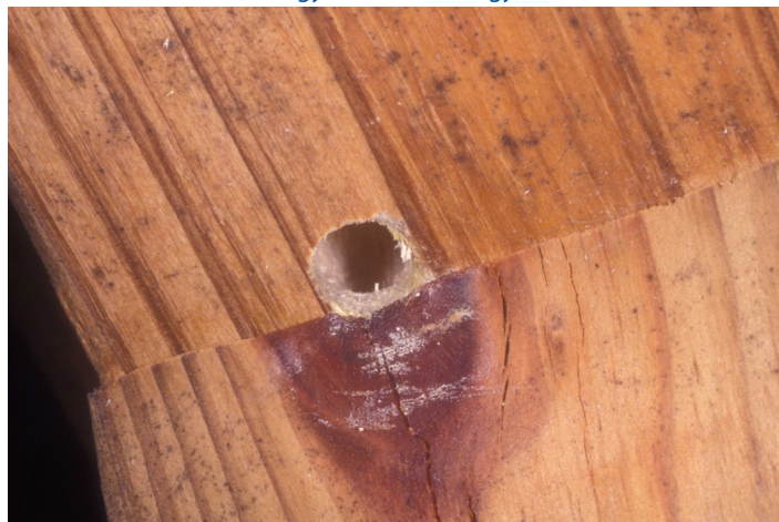
Figure 4. Carpenter bee damage to mailbox.
