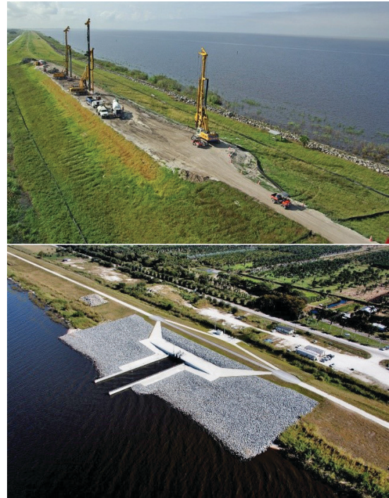
Figure 5. The US Army Corps Herbert Hoover Dike Rehabilitation Project, begun in 2007, includes installation of concrete cut-off walls in the center of the earthen dike (top photo) as well as repair or replacement of the inflow/outflow structures (bottom photo). Credits: US Army Corps of Engineers
